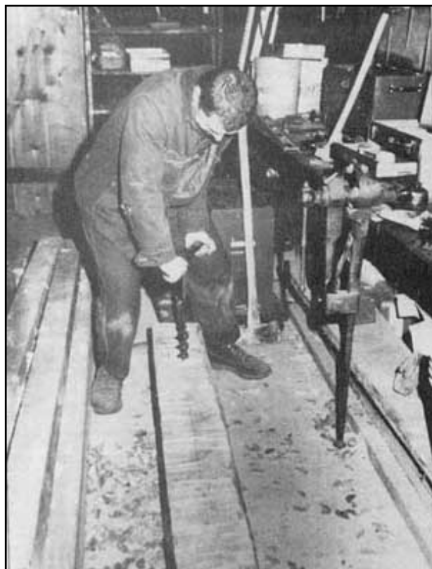
Pictures 8 and 9. Using the template in Diagram 3, draw the top lines and drill the holes.
