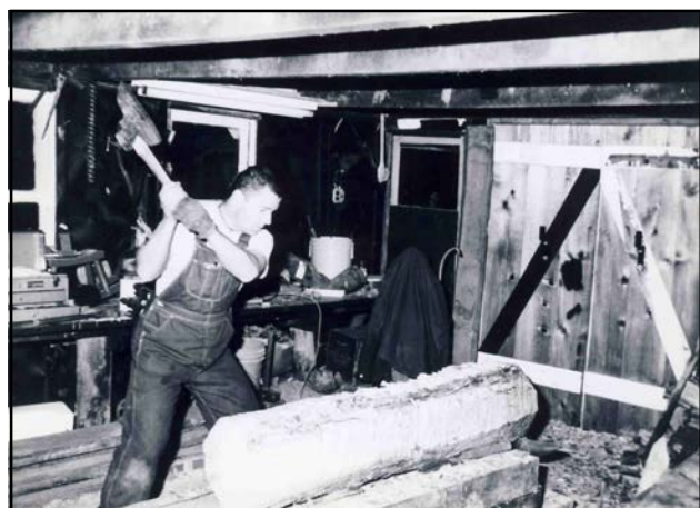
Picture 2. Here I'm using a broad ax to hew the log.
