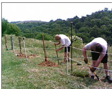
Tulsi and Nirguna digging holes for fence posts
