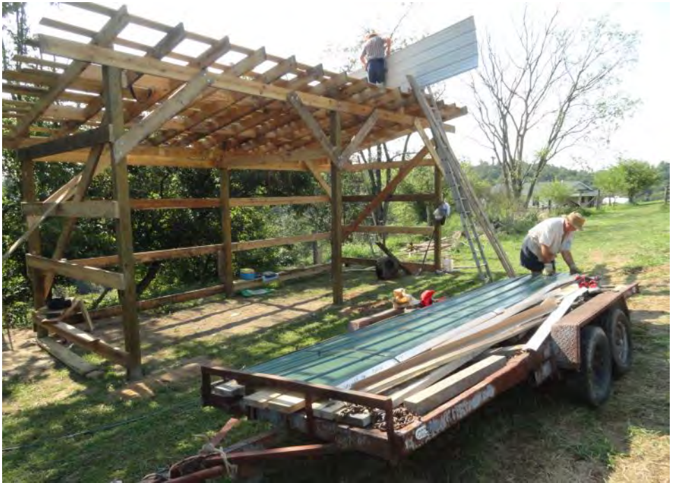
Mike (on the ground) and John (on the roof), working towards finishing the roof. Roofing material was 3 feet wide and 16 feet long. In the photo to the right you can see the finished shelter with its 1 x 6 poplar siding in place. The nails used for the building were all galvanized so there will be no rust. The siding was painted with clear "Dura-Coat."
