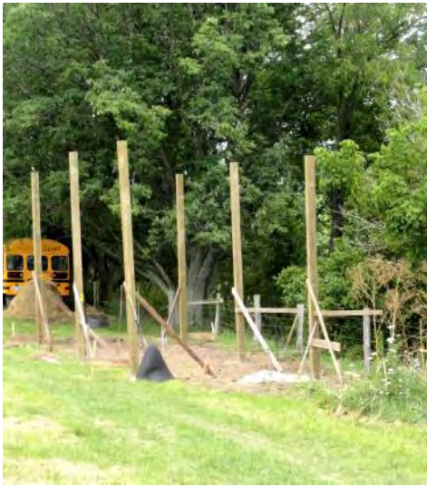
Above: 6 x 6 uprights in place. Below: Horizontal bracing in place and roof going up.
