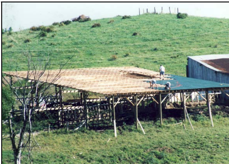
Top: Mike securing nailers for the new tin roof on the barn.
