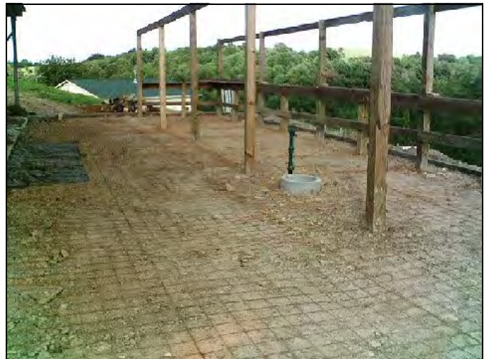
Right: The support beams for the extended roof were put in place. Then wire mesh was placed over the shale as a reinforcement for the cement floor. A water hydrant was placed in the middle of the floor.
