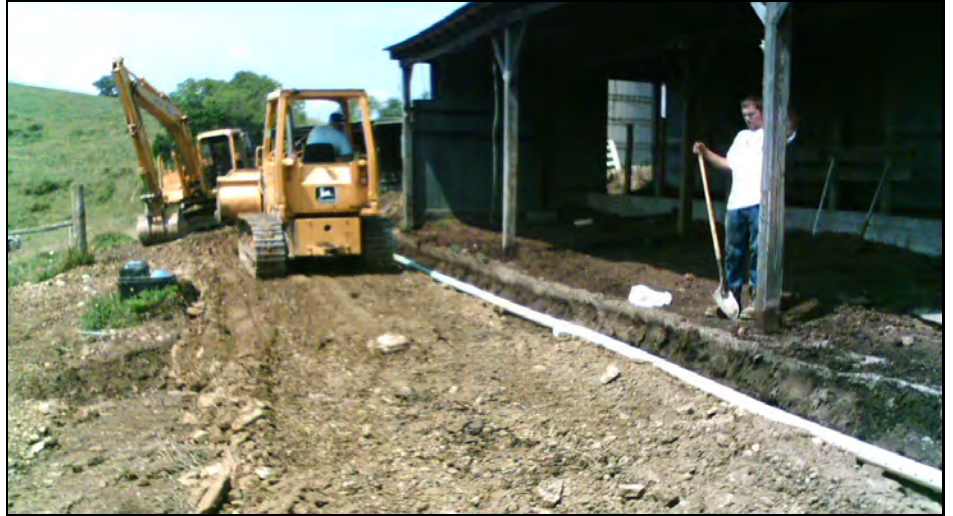
Top: The work site was excavated down to virgin soil and the new French drain was installed.
