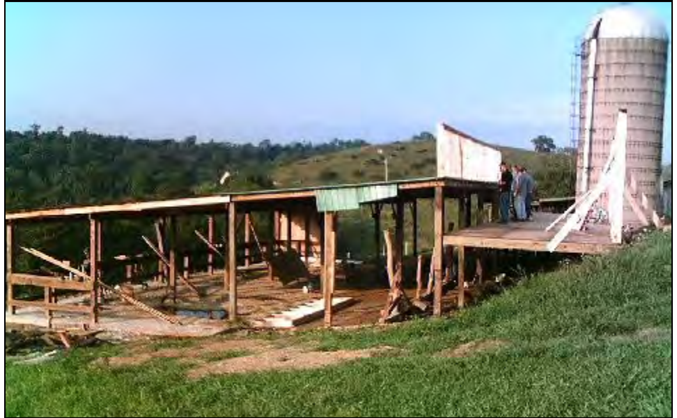
Top: The hay storage deck is in place and walls are being framed.
