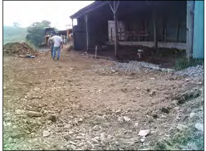
Right Middle: The excavated site was then backfilled with shale.
