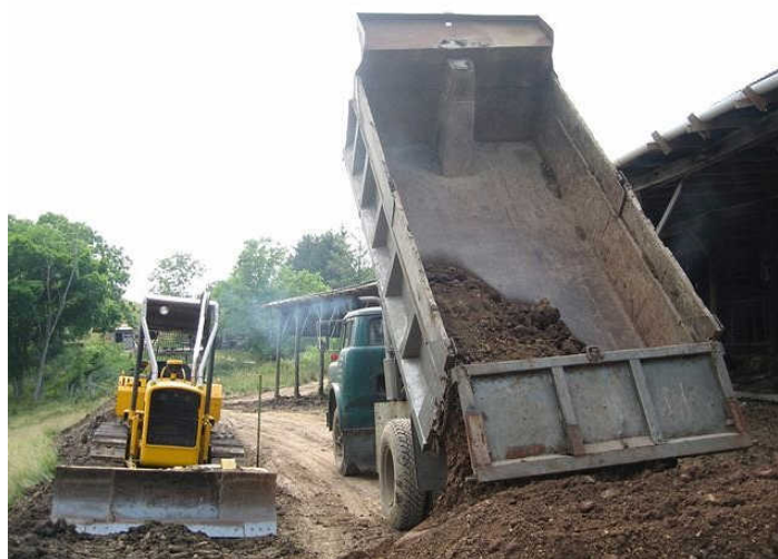
Dumping and spreading the dirt fill in front of the barn before laying wire mesh and then pouring concrete.
