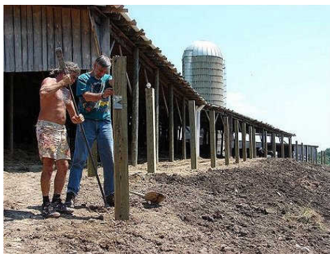
Installing fence line and new barn poles.
