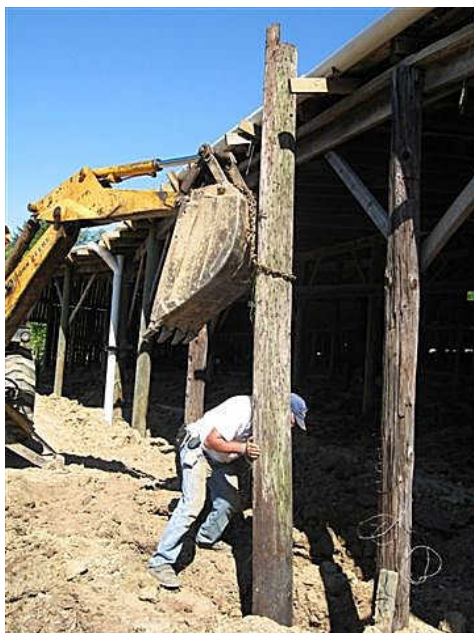
Installing fence line and new barn poles.
