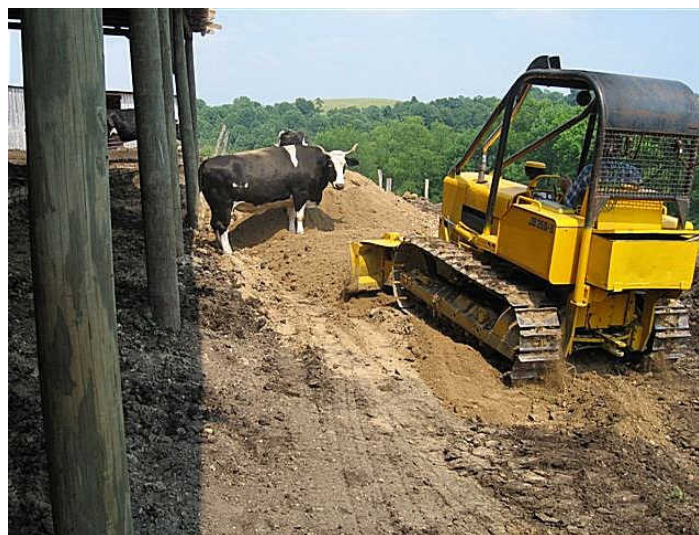
Dumping and spreading the dirt fill in front of the barn before laying wire mesh and then pouring concrete.
