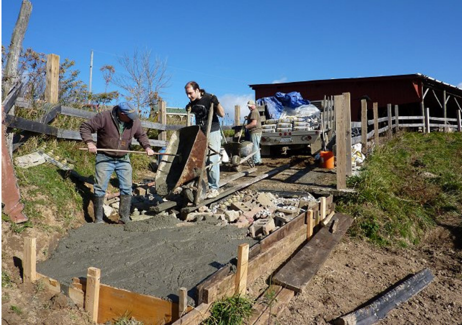
Vaisnava delivers a load of concrete to Balabhadra while Janardan mixes his next load.
