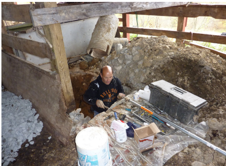
Tejo , our plumber, getting everything ready to install the new frostless water hydrant.
