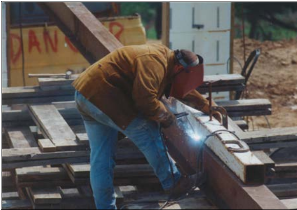
Right - Baladeva welding two steel beams together to form the support beam for the next two floors.
