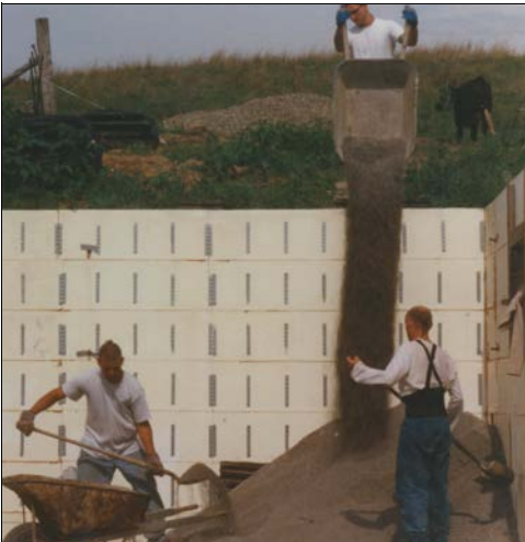
Left- Moving 33 tons of sand onto the basement floor with wheelbarrow and shovel.
