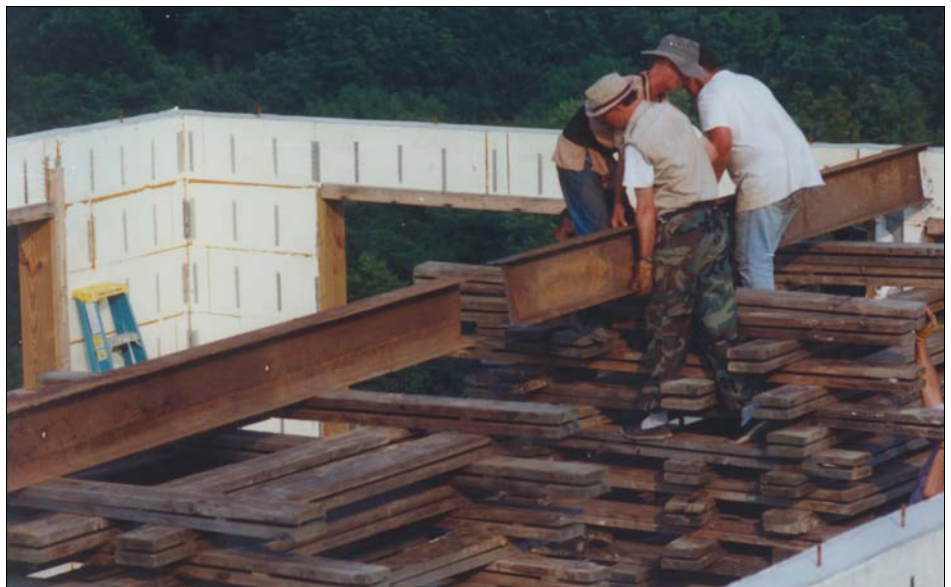
Bottom - Raising the steel I-beams that will help to support the next two floors.
