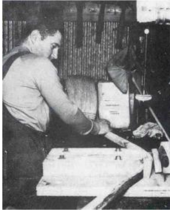
Here is how the steamed bow stick is bent on the form.
