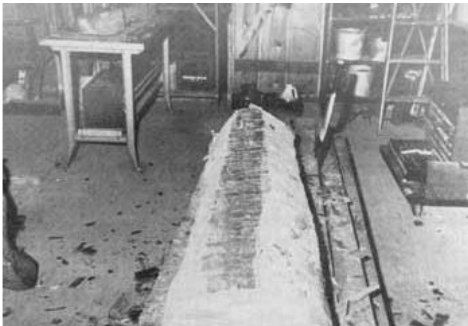
Picture 3. Continue hewing the log until it's squared out.
