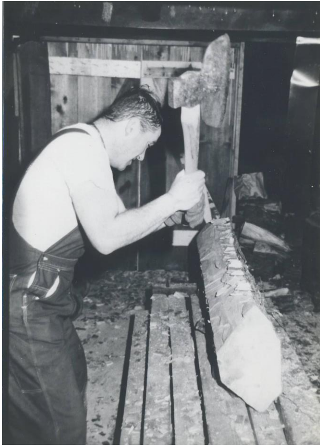
Picture 4. Beginning to square the log.
