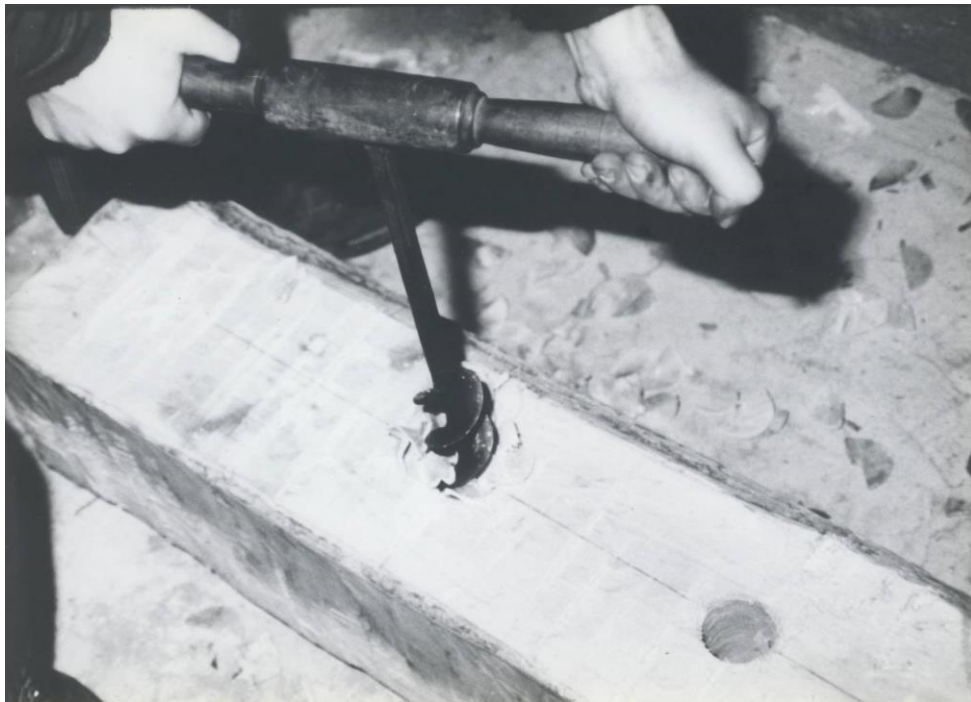
Picture 10. A hand auger is a simple way to drill the two inch holes.
